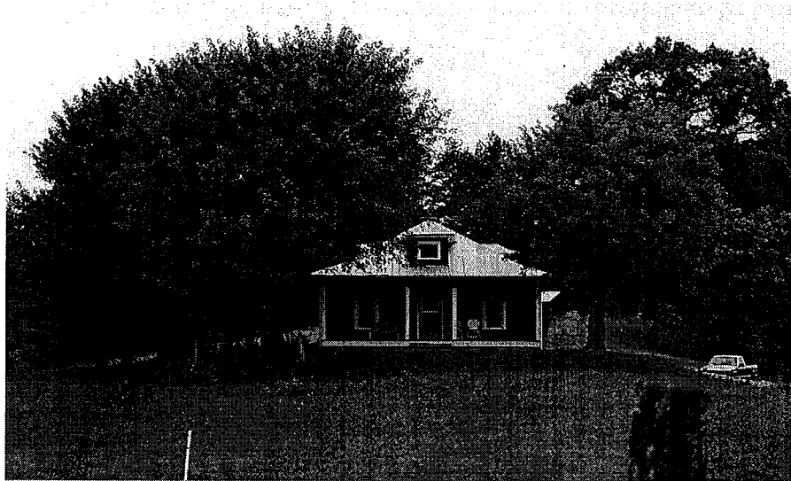
Figure 37. Property 30 - House. The house has been determined not eligible for the National Register because it is neither historically nor architecturally significant. Photographed July 26, 2000.
