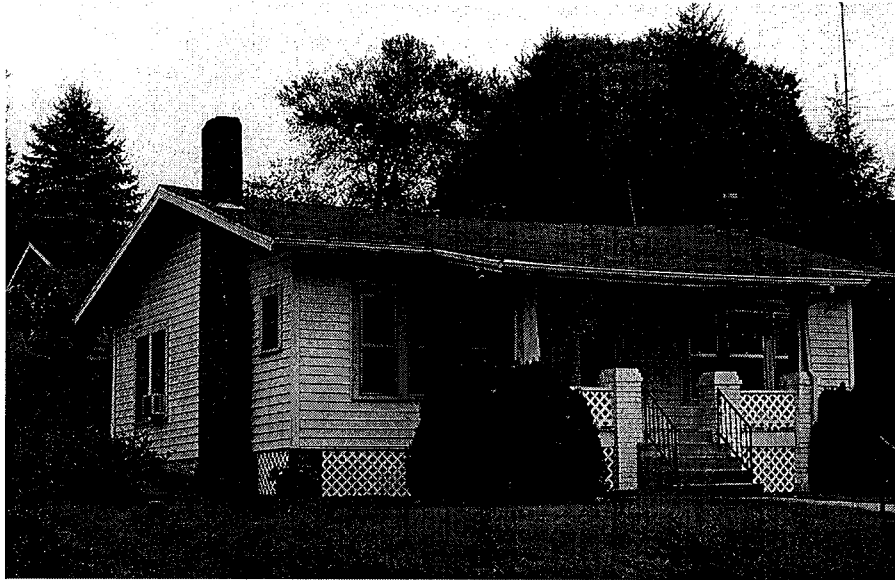
Figure 34. Property 27 - House. The house has been determined not eligible for the National Register because it is neither historically nor architecturally significant. Photographed July 26, 2000.
