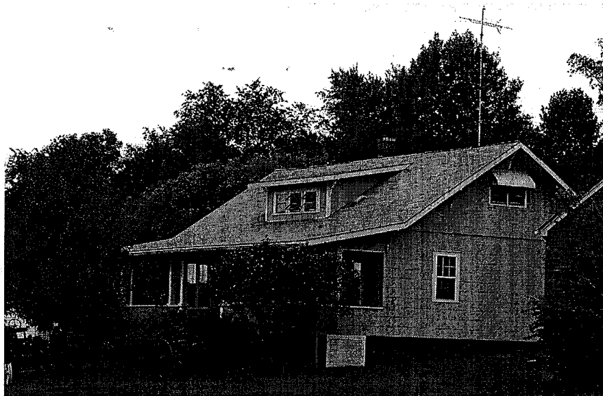
Figure 35. Property 28 - House. The house has been determined not eligible for the National Register because it is neither historically nor architecturally significant. Photographed July 26, 2000.
