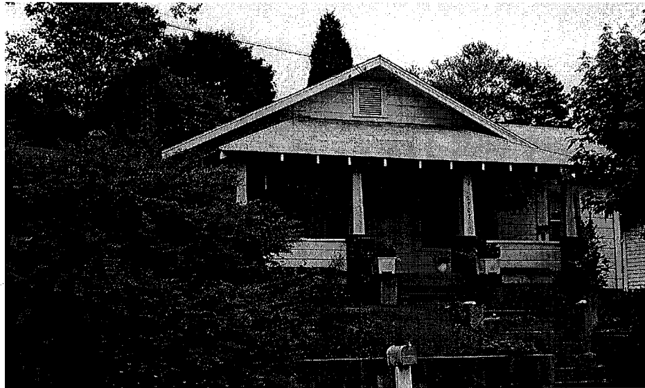
Figure 33. Property 26 - House. The house has been determined not eligible for the National Register because it is neither historically nor architecturally significant. Photographed July 26, 2000.
