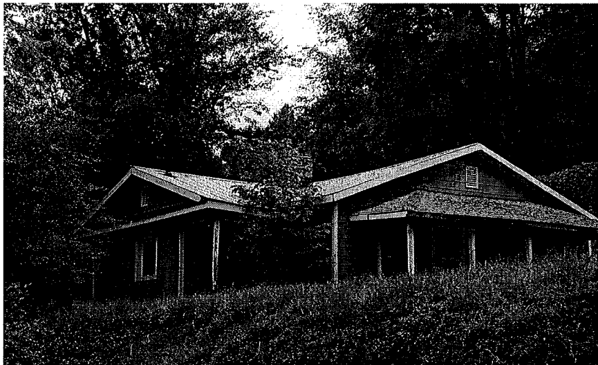
Figure 29. Property 5 - House. The house has been determined not eligible for the National Register because it is neither historically nor architecturally significant. Photographed July 26, 2000.
